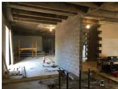
First floor looking west
