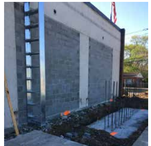
Front of building with bays walled off
