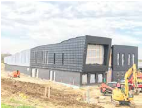
Front of Building
