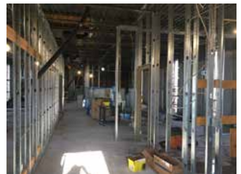
Second floor looking west
